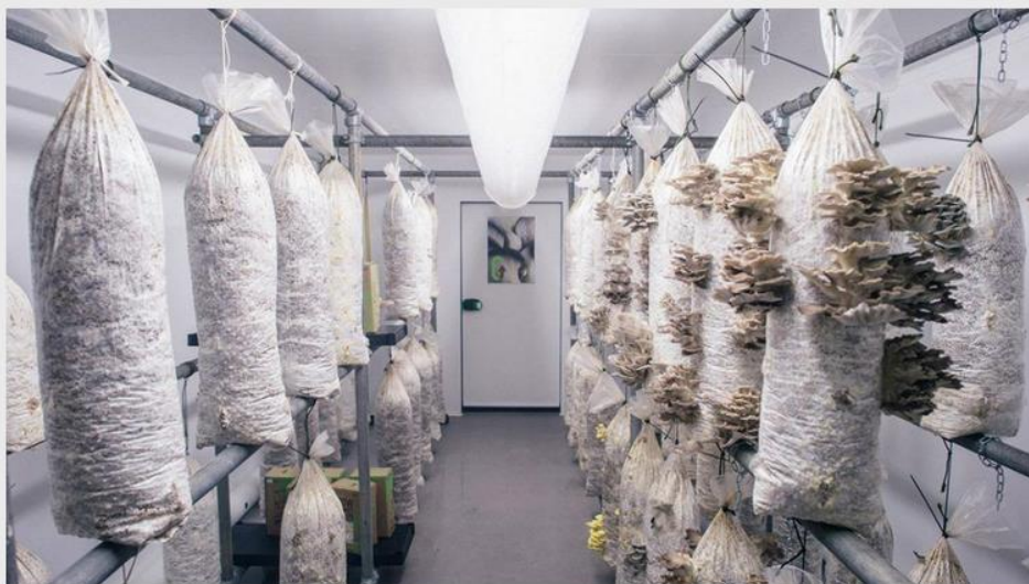
Insulated fridge panel room - providing a well insulated and sealed space, GroCycle Urban Mushroom Farm
