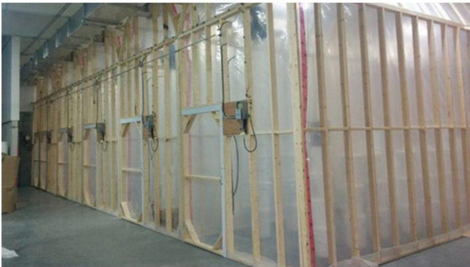
Wooden stud frame with plastic sheeting, Blanc de Gris Mushroom Farm in Montreal
